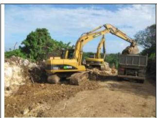
Widening the road near La Cressonniere Ranch. An hydraulic rock breaker (middle background) chips out the coral while another excavator loads the excavated material into a truck.
