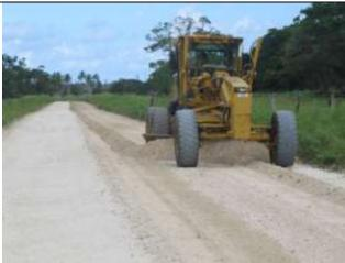
A Downer EDI Works grader carrying out a maintenance grade on the existing unsealed road between Eton and Rentabo so that a smooth surface for traffic is restored after the recent rain.
